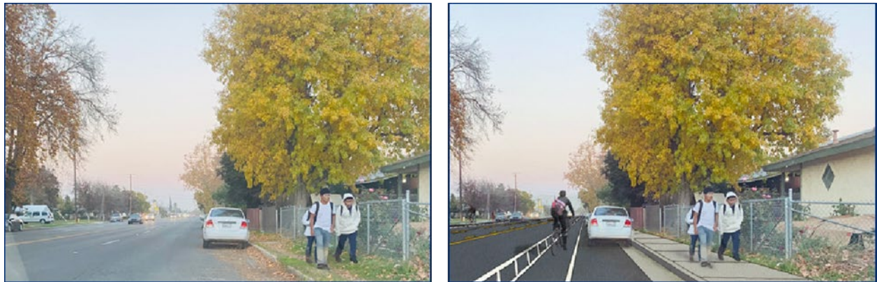
Examples of complete streets policy implementation by Caltrans. Bike Lanes on SR 145 at Yosemite Ave Between Lyons St & Mace St: Existing Design (left) vs. Proposed Design (right)
