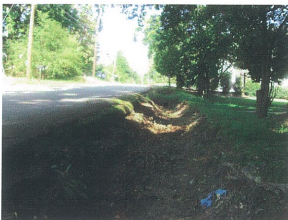
Figure 10. Dangerous ditch that parallels Church Street extremely close to the edge of pavement.
