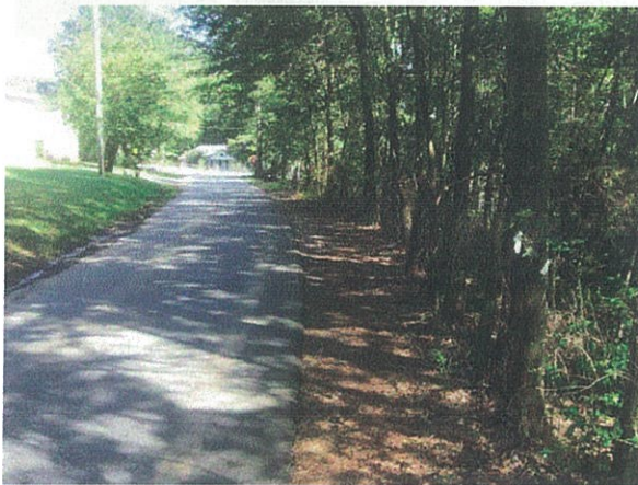
Figure 8. Jones Road, looking East. Road carries two-way traffic and is only 12ft. in width. Water has begun ponding on the North side of the road.
