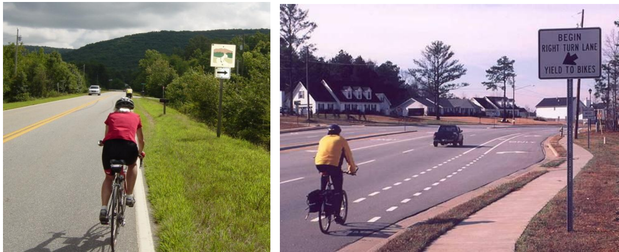
a) Bicycle route, Scenic Byway, N. Georgia; b) Bicycle lane, Sugarloaf Parkway, Gwinnett County
