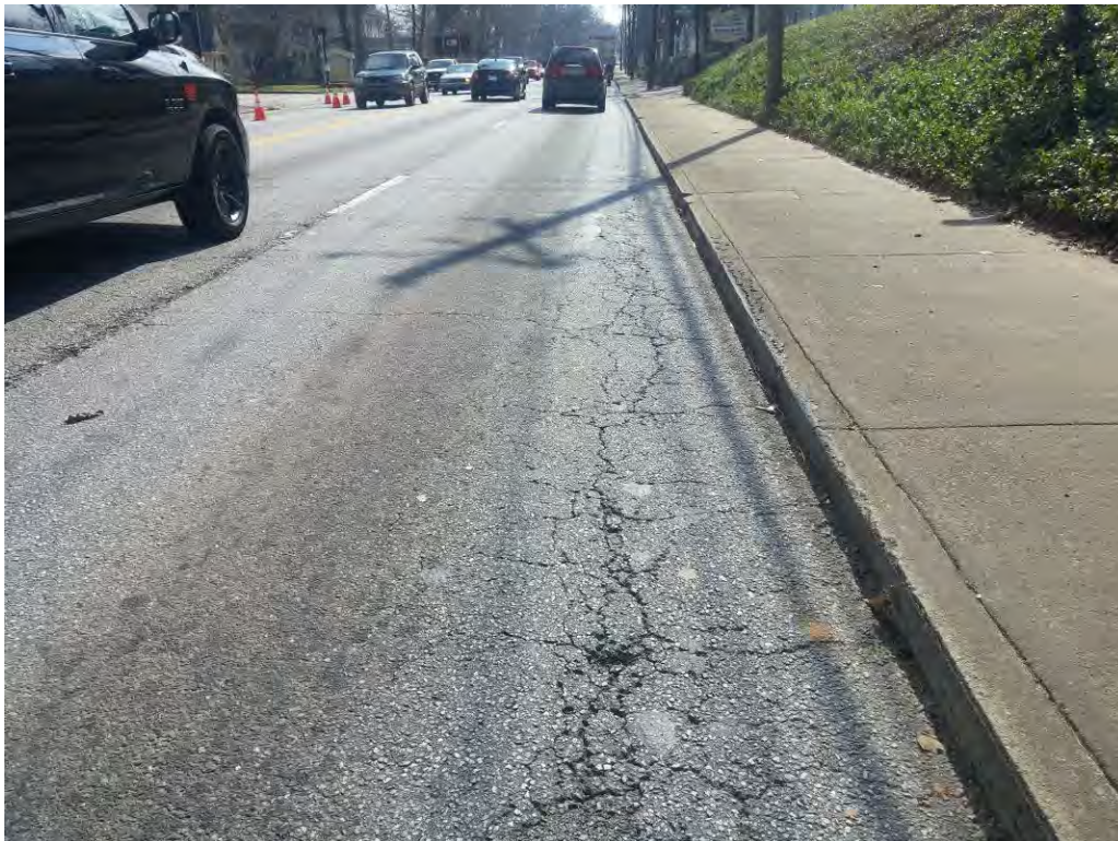
Load Cracking Level 3, SR 11, Station 9 + 00, SB, Lane 2
