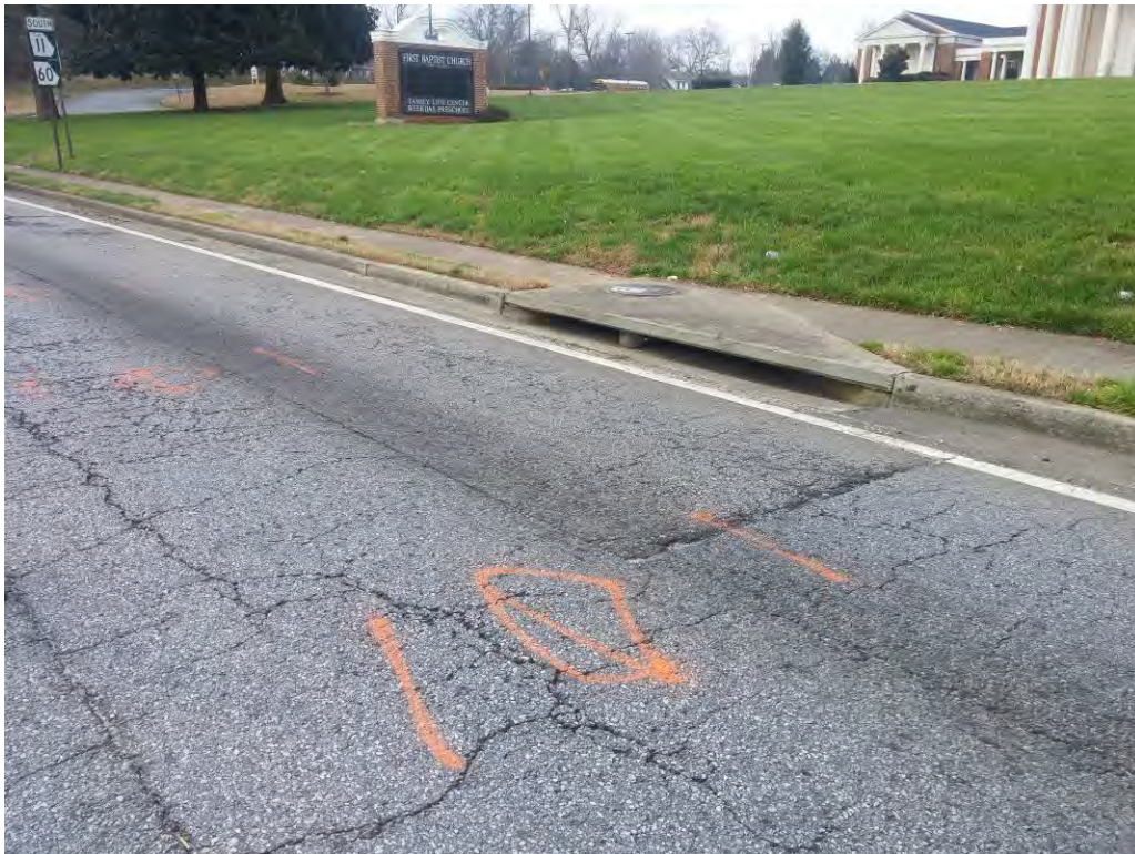
Block/ Transverse Cracking Level 2, SR 11, Station 4 + 00, SB, Lane 2
