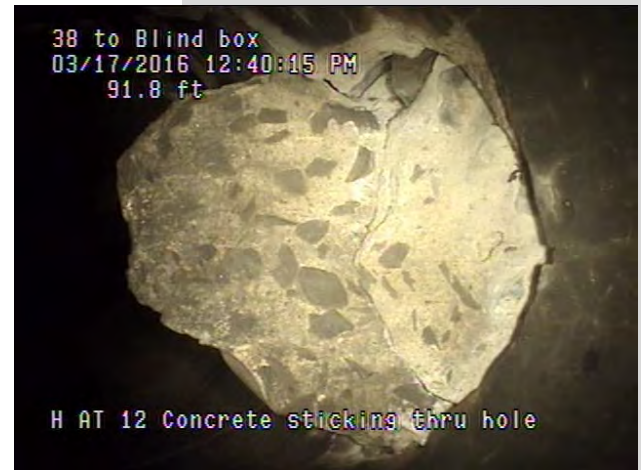
CONCRETE INTRUSION
