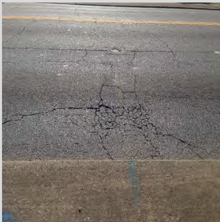
EXAMPLE OF PAVEMENT CRACKING
