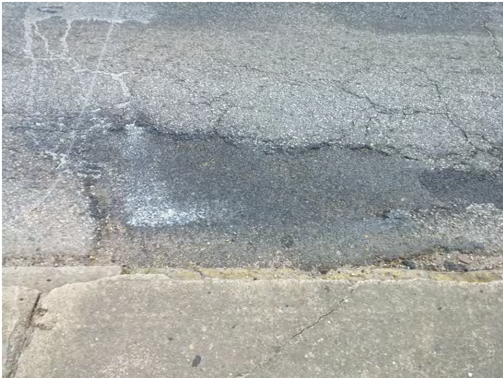
Potholes associated with Level 4 Load Cracking, Station 15 + 00, SB, Lane 2
