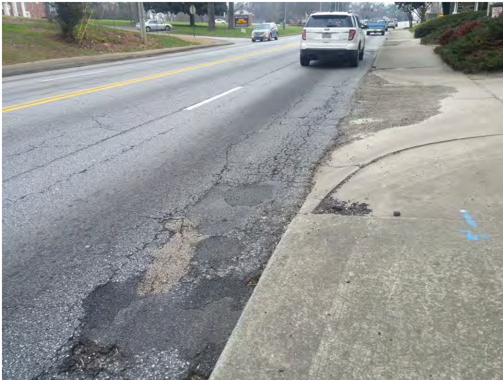
Patches associated with Load Cracking Level 3, SR 11, Station 7 + 00, NB, Lane 2
