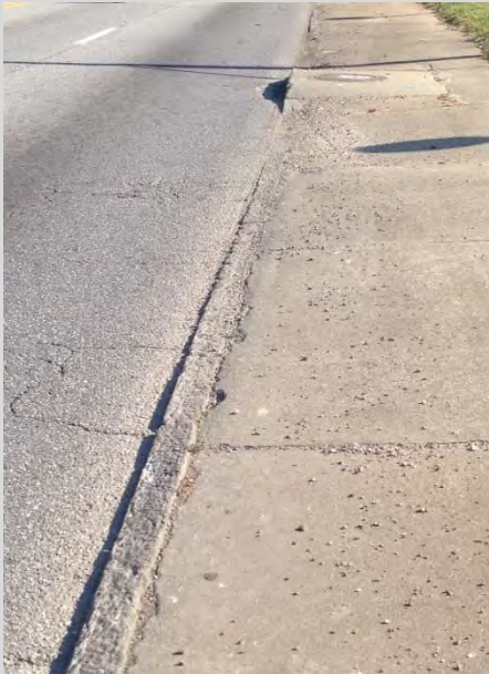
EXAMPLE OF AREA WHERE TOP OF CURB AND PAVEMENT ARE LEVEL
