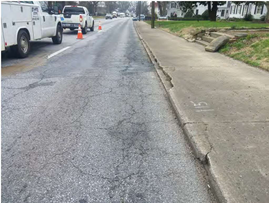
Load Cracking Level 3, SR 11, Station 15 + 00, SB, Lane 2
