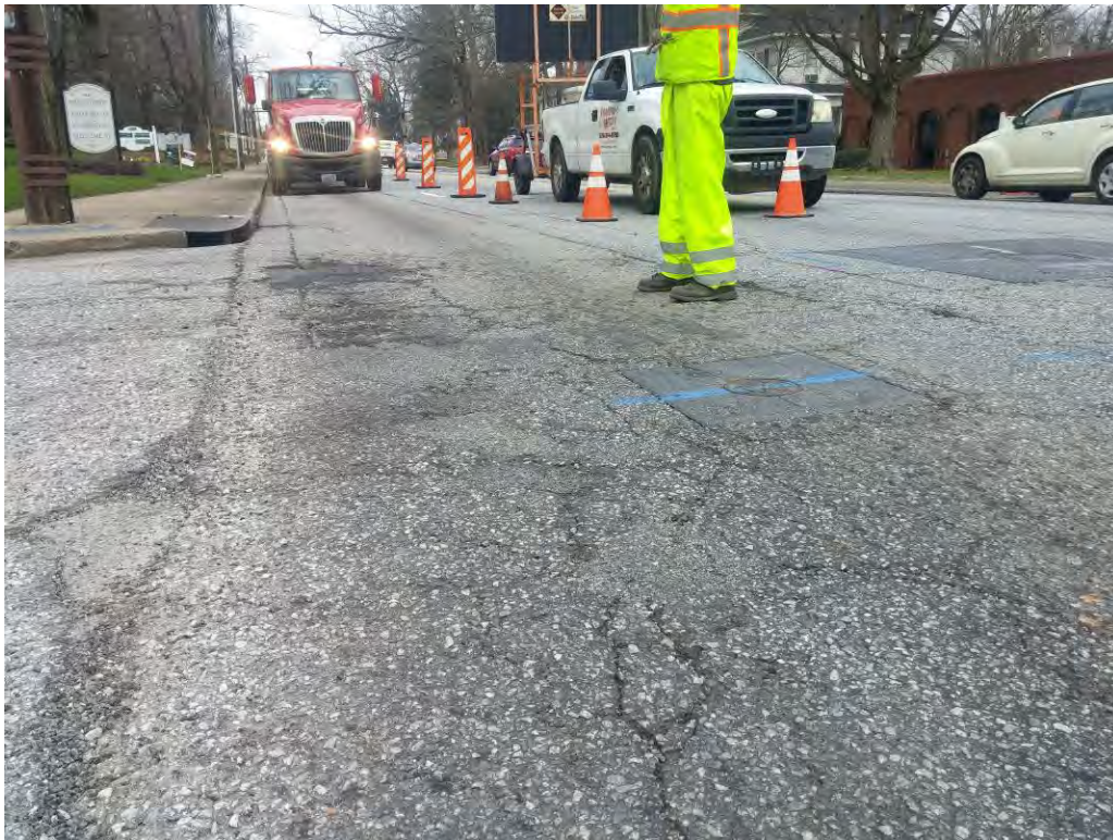
Raveling Level 2 and Load Cracking Level 4, SR 11, Station 15 + 00, SB, Lane 2
