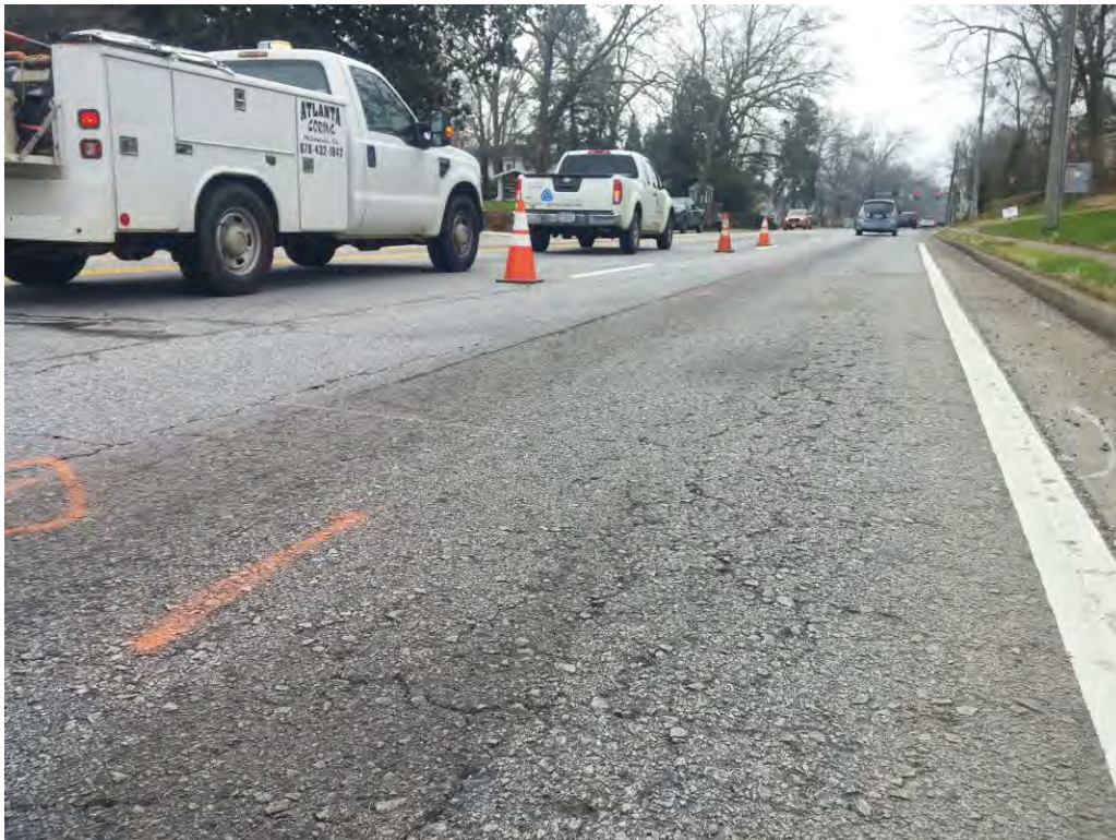
Raveling Level 2, SR 11, Station 4 + 00, SB, Lane 2
