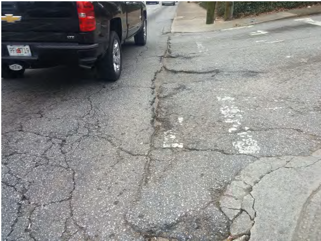
Edge Distress Level 2, SR 11, Station 11 + 00, Southbound, Lane 2
