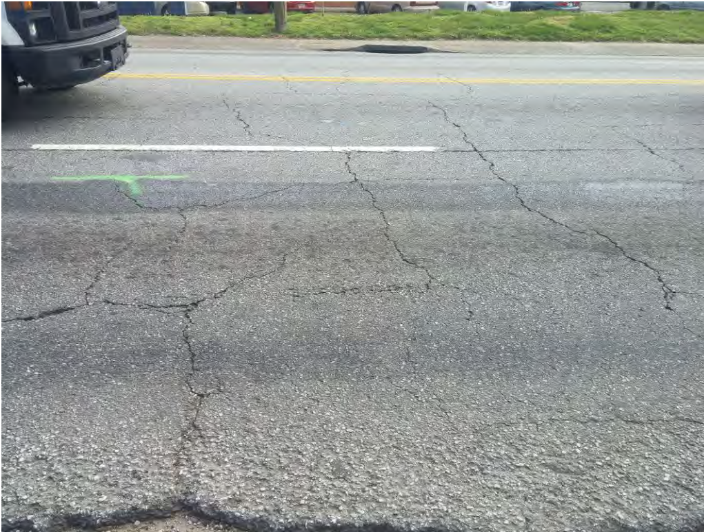
Block/ Transverse Cracking Level 2, SR 11, Station 15 + 00, SB, Lane 2
