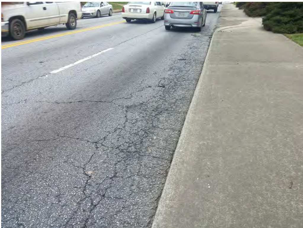
Load Cracking Level 4, SR 11, Station 18 + 00, SB, Lane 2
