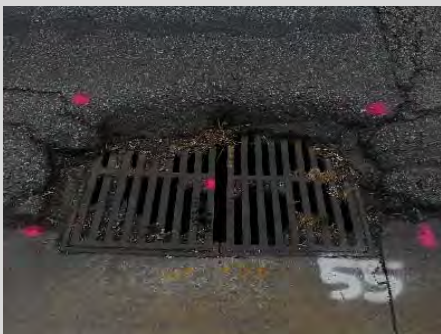
INLET PARTIALLY COVERED BY ASPHALT AND INACCESSIBLE
