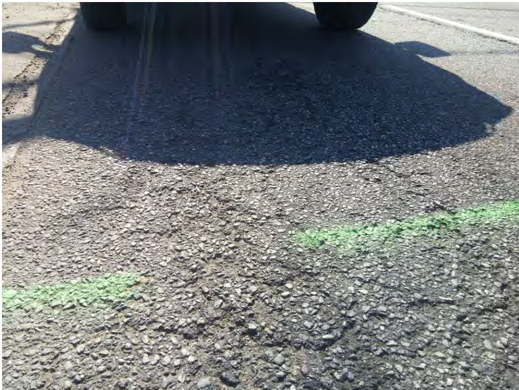
Raveling Level 2, SR 11, Station 26 + 00, SB, Lane 2
