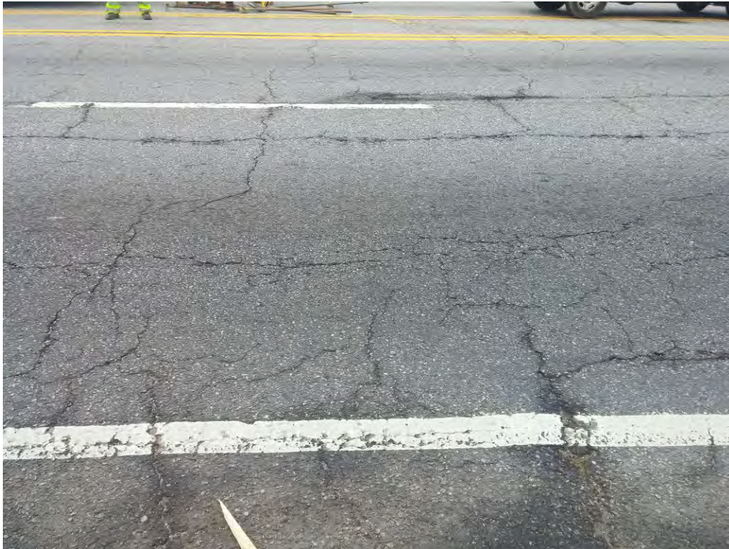
Block/ Transverse Distress Cracking Level 1, SR 11, Station 4 + 00, NB, Lane 2
