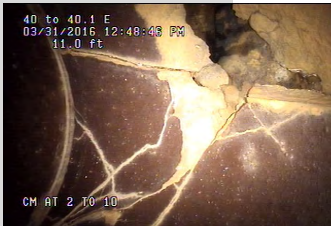
EXAMPLE OF COMMONLY FOUND CRACKED CLAY PIPE
