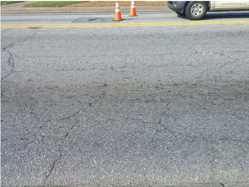
Block/ Transverse Cracking Level 1, SR 11, Station 15 + 00, NB, Lane 1
