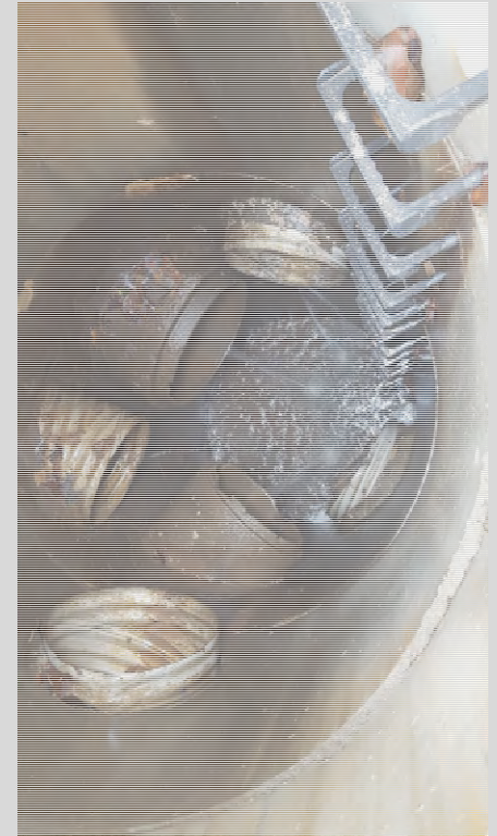
MULTIPLE PIPE CONNECTIONS NEAR OUTFALL BEHIND THE TIMES BUILDING
