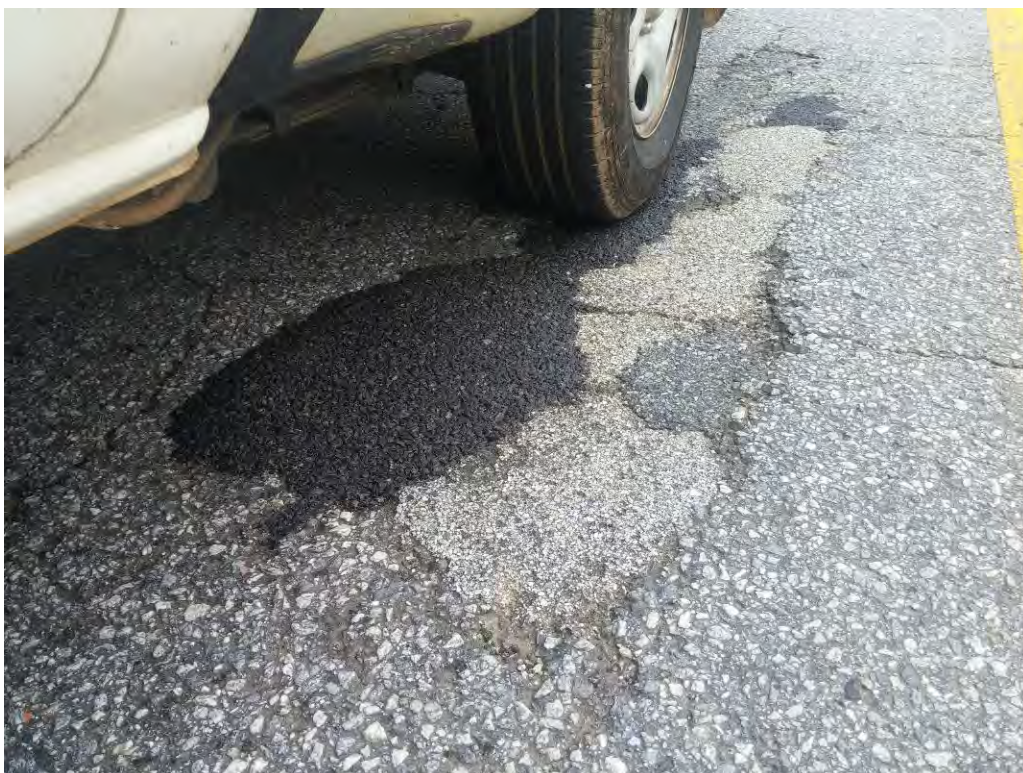
Potholes/Patches, SR 11, Station 15 + 00, SB, Lane 1
