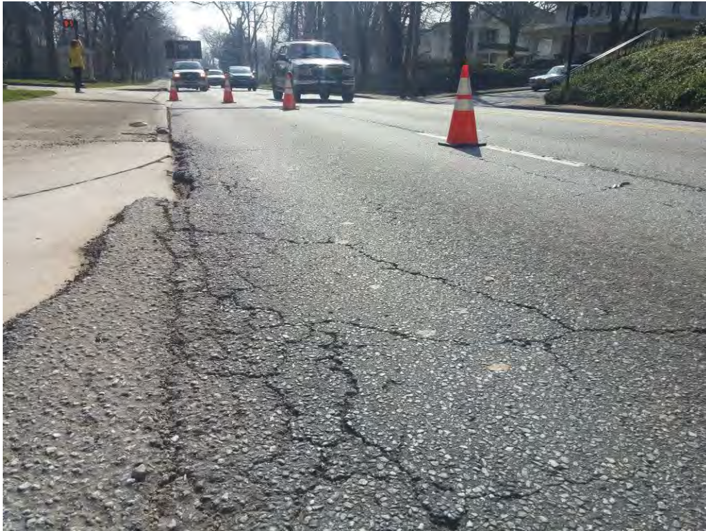
Edge Distress Level 3, SR 11, Station 9 + 00, Northbound, Lane 2
