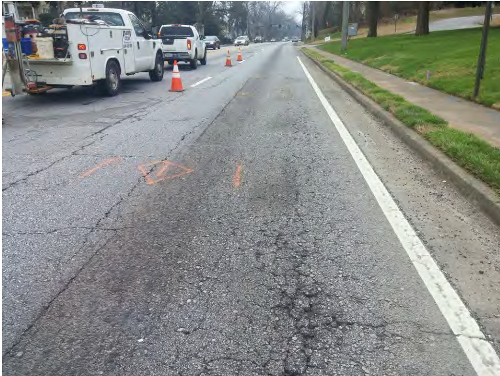
Load Cracking Level 3 – SR 11, Station 4 + 00, SB, Lane 2
