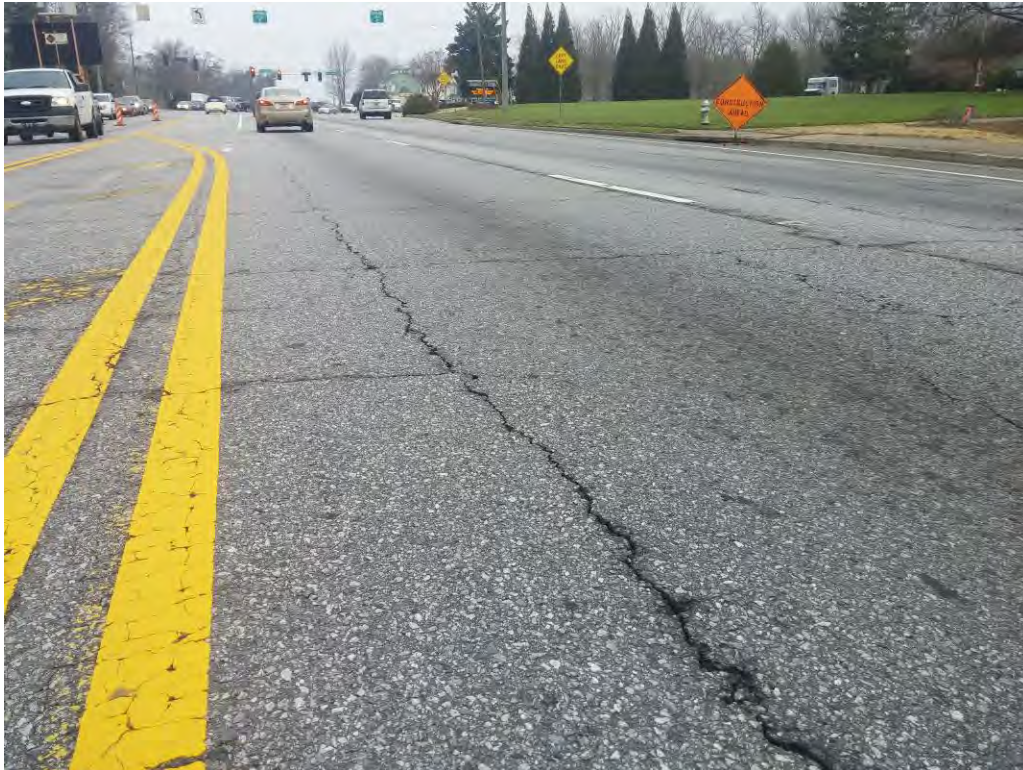
Load Cracking Level 1 – SR 11, Station 4 + 00, NB, Lane 1
