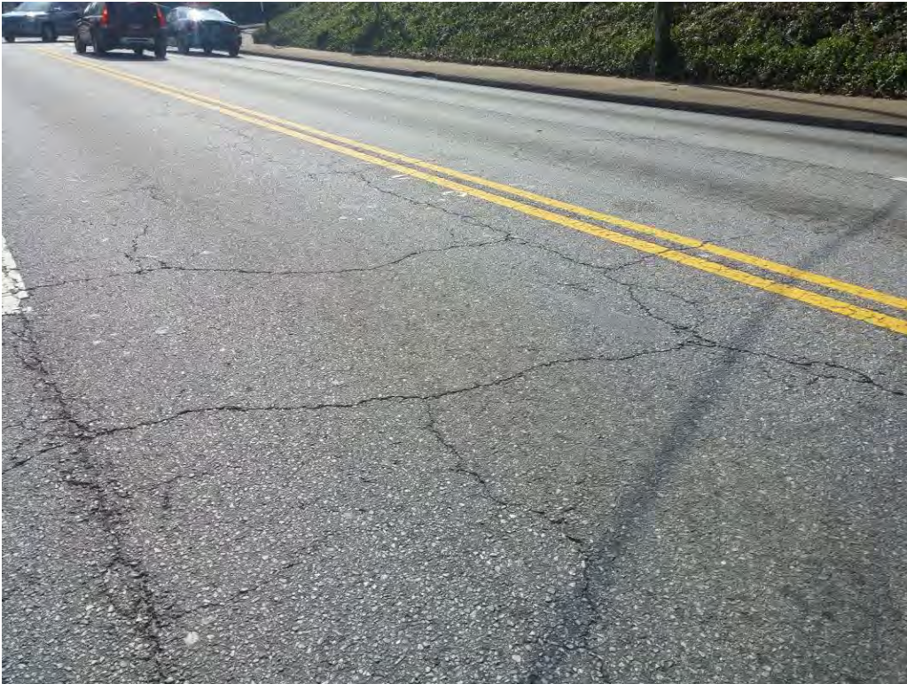
Block/ Transverse Cracking Level 2, SR 11, Station 9 + 00, NB, Lane 1
