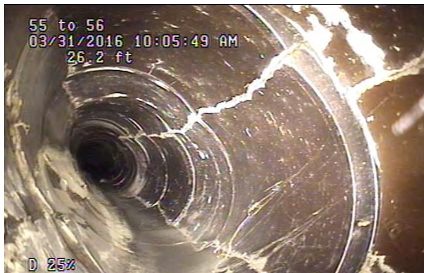
EXAMPLE OF EGGED CLAY PIPE COMMONLY FOUND ALONG CORRIDOR
