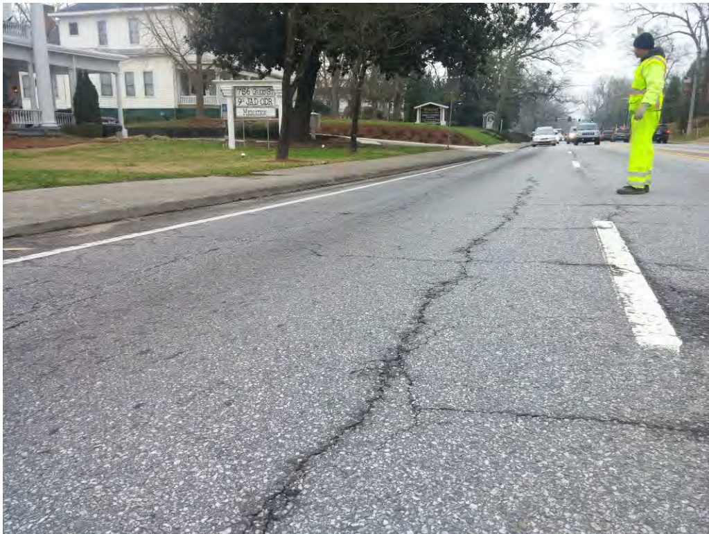
Load Cracking Level 1 – SR 11, Station 4 + 00, NB, Lane 2
