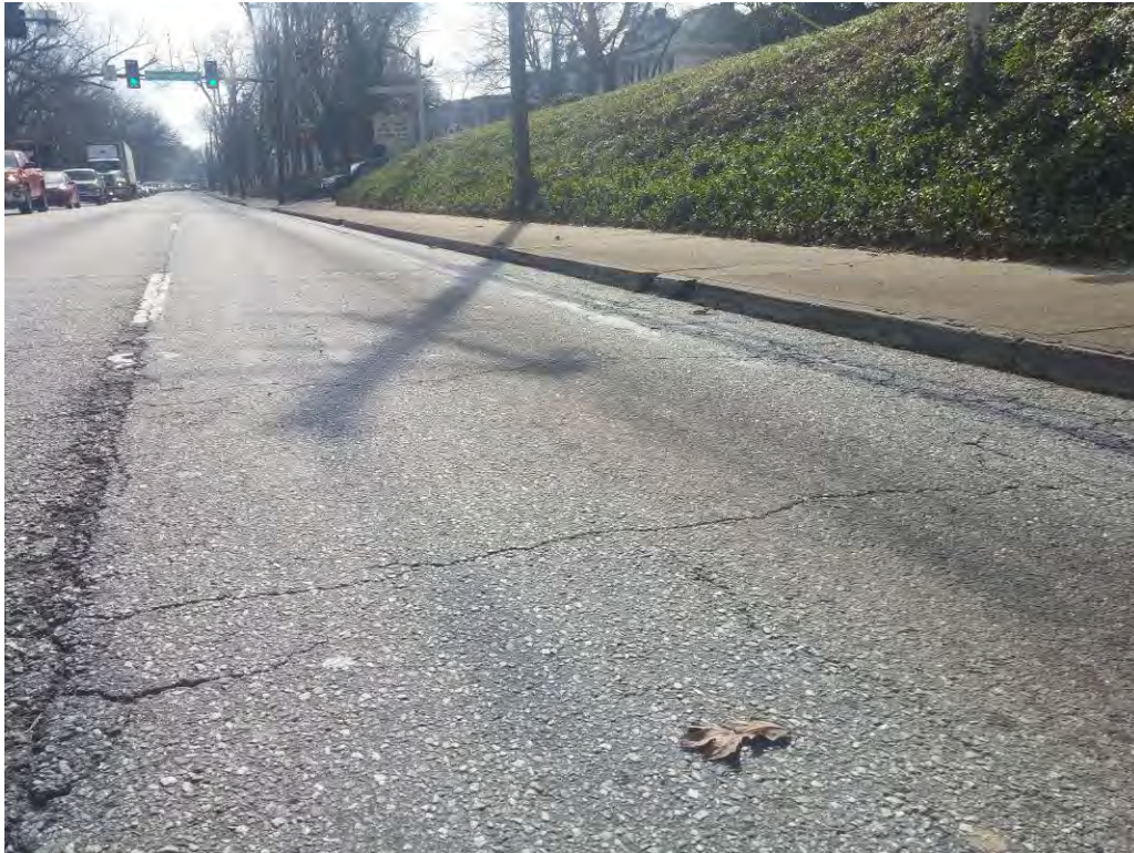
Raveling Level 1, SR 11, Station 9 + 00, SB, lane 2
