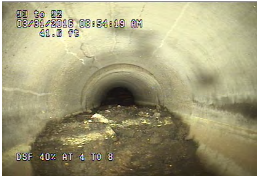
EXAMPLE OF PIPE PARTIALLY BLOCKED BY DEBRIS
