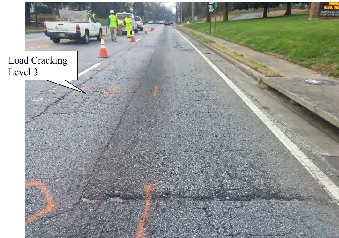
Raveling Associated with Load Cracking Level 3, at Station 4 + 00, SB, Lane 2
