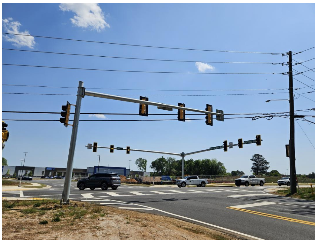
Figure 4.3 – SR 53 at Peachtree Road Intersection
