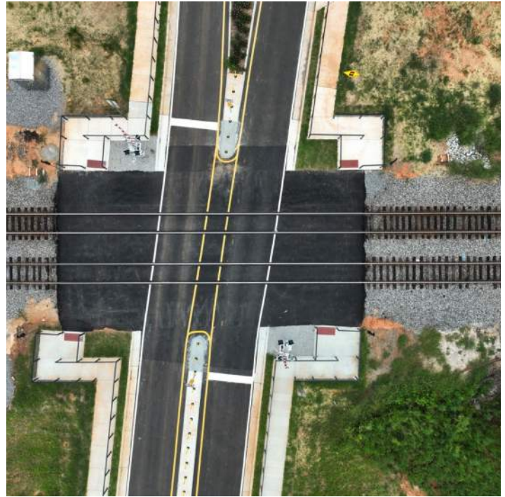
Z-Gate Railroad Crossing example
