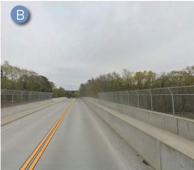
The Tumbling Creek Road bridge (over the railroad) was recently replaced, and was built with a 10’ sidewalk which can serve as a link for the Highlands to Islands trail system.
