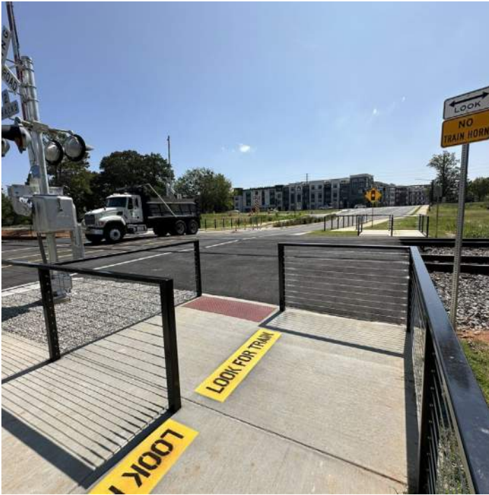
Z-Gate Railroad Crossing example
