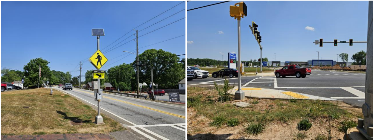
Figure 2.8 – Existing Pedestrian Infrastructure (Left: Rectangular Rapid Flashing Beacon in front of the City Hall; Right: ADA ramps at SR 53 and Peachtree Road intersection without sidewalk connection)
