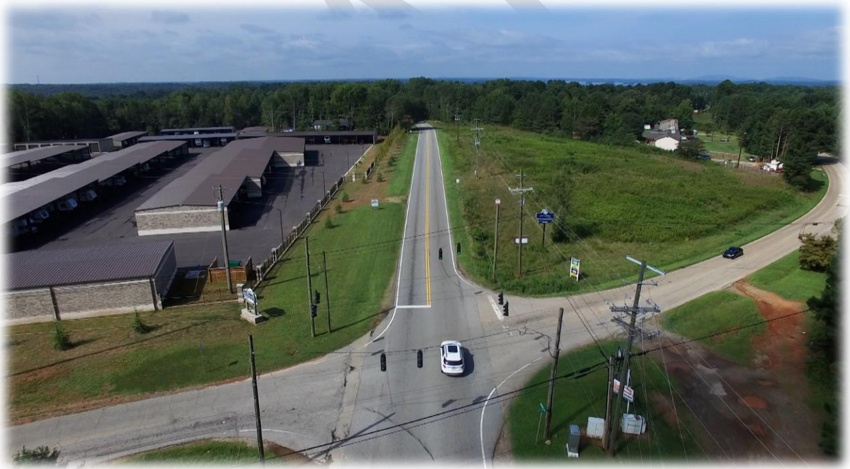
McEver Road at Lights Ferry Road, the site of a new roundabout opening in 2027.
